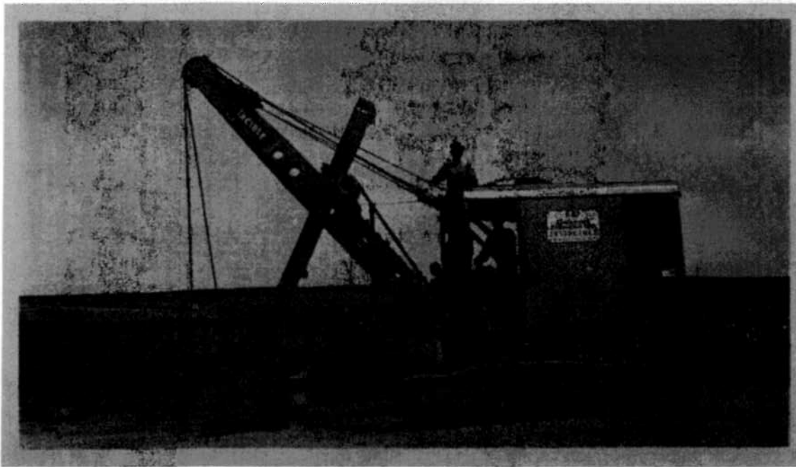
Civilian Conservation Corps crew using a dragline on a refuge.
